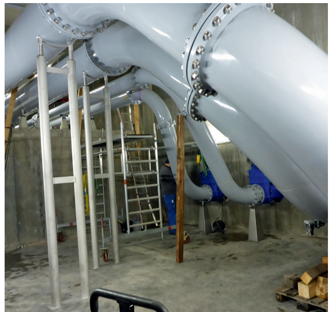
Source: Customer photo during installation
